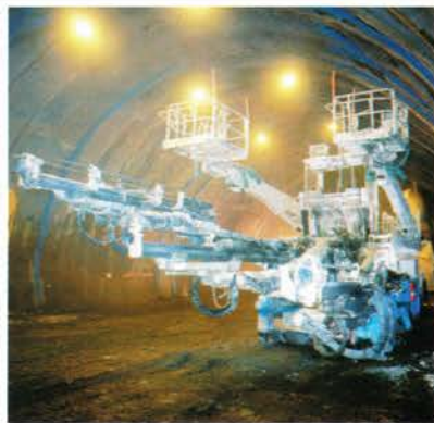
Tunnel Drill Jumbo
