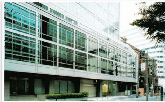
Furukawa Osaka Building (Osaka Prefecture)
