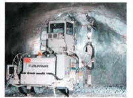
Tunnel Drill Jumbo
